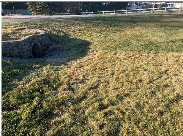
29 Gundalow - 1 (Drainage Area)
