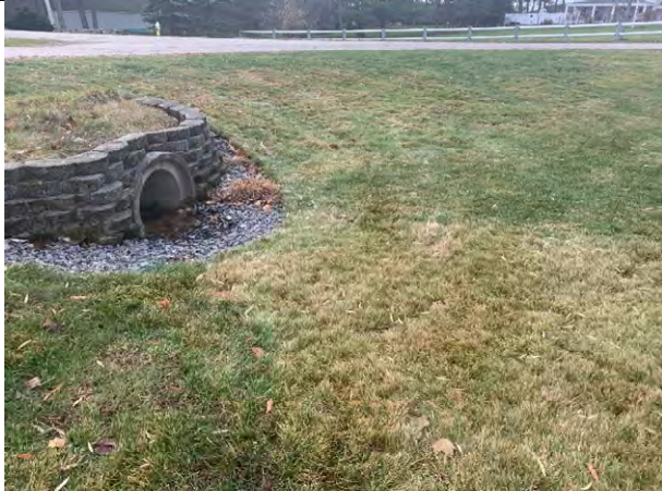
29 Gundalow - 1 (Drainage Area)
