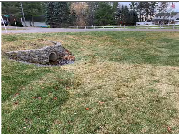
29 Gundalow - 1 (Drainage Area)
