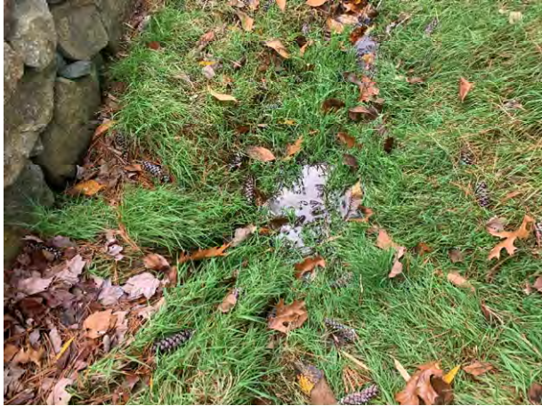
4 Brickyard Circle – 3 (Drainage Course)
